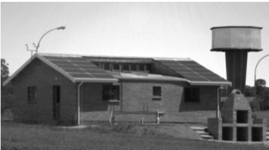
Langalinamandla, the energy efficient grid-independent solar house with solar panels and solar water heater panels on the north facing roof
