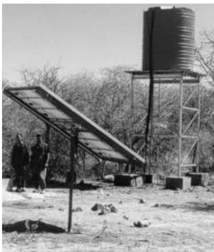
Solar energy water pump (photo: Robert Schultz)
