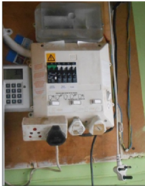
Figure 3: Prepayment electricity meter shared between the owner/seller and three other households buying electricity connected by an extension cord [5]
