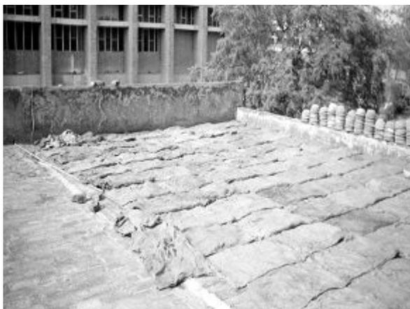
**Figure 1: Roof treated with sacks filled with sawdust**
